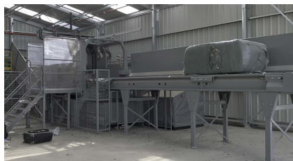
> High capacity bale opening ensures steady fuel intake.
